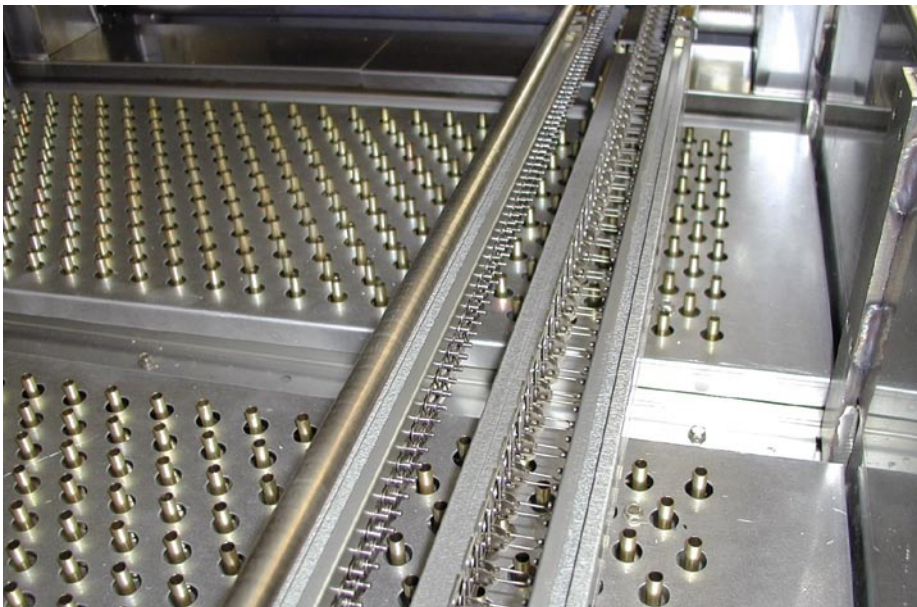
Center support and conveyor
